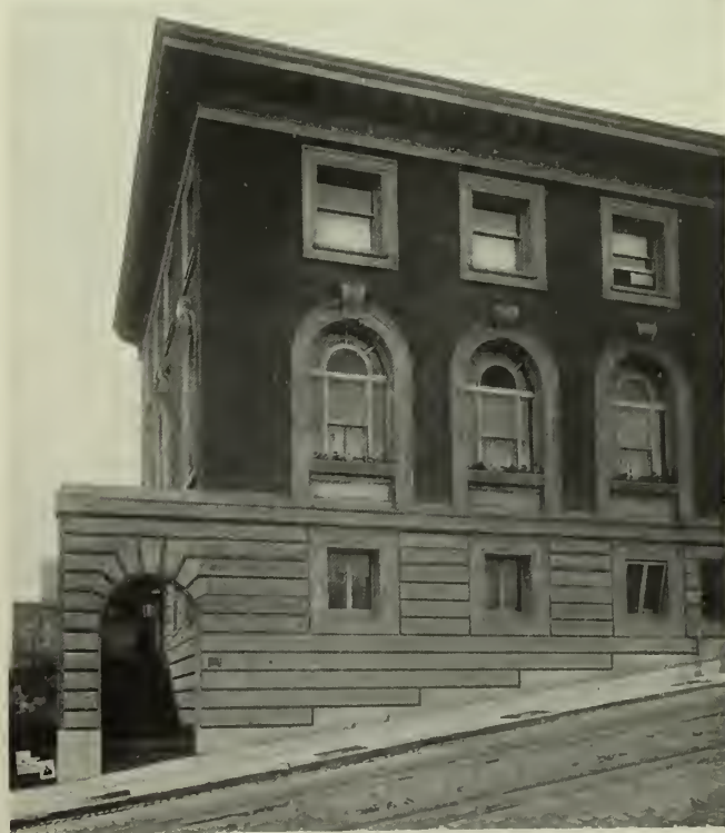
ENTRANCE TO THE FAMILY CLUB. C. A. Meussdorffer, Architect.
